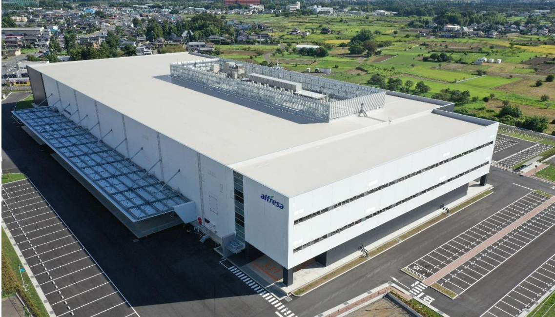
Exterior View of the Tsukuba Distribution Center
